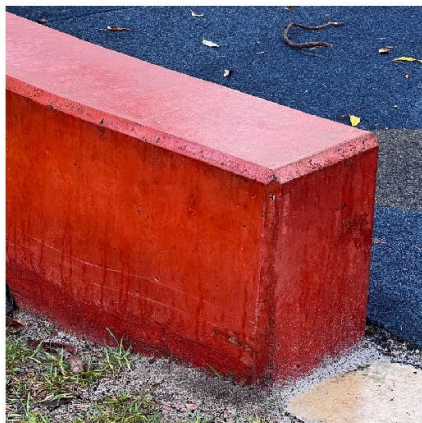
Formed concrete seating walls
